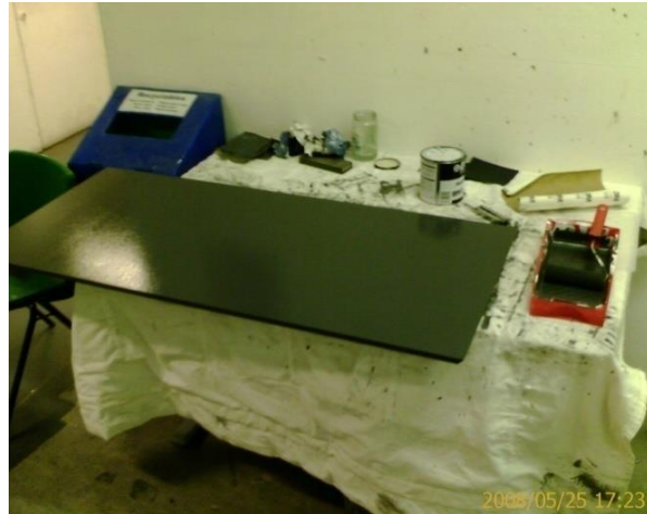
Figure 31: A satin-based top coat provides colour. A clear varnish was applied to aid durability.
